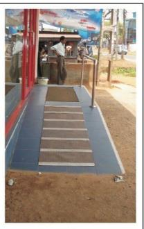
Ramp surface This picture shows an adjustment that was made to a ramp because the surface was too slippery. Ramp surfaces that are too slippery are very dangerous for people with and without disabilities and can cause serious falls. There is good colour contrast on the edge of this ramp but there are no handrails.
